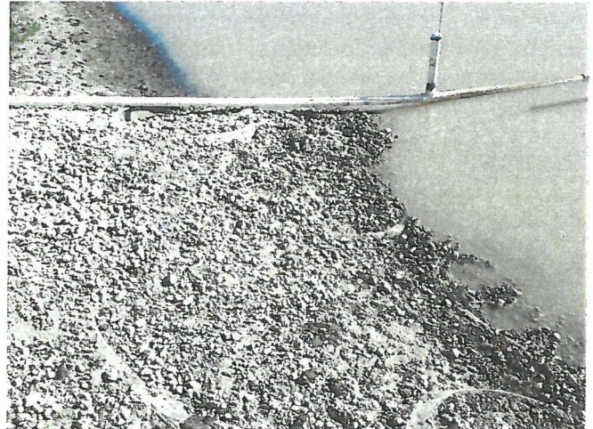
Figure #2 Open top tire mat with gravel fill on a geotextile base.
